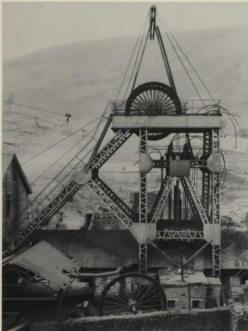
Winding Tower, Park Colliery, Treorchy, South Wales
