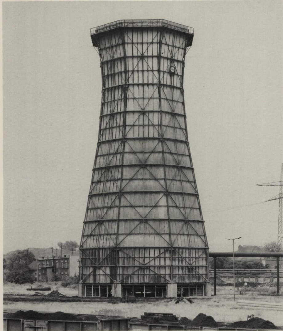
Cooling Tower, Concordia Colliery, Oberhausen, Ruhrdistrict
